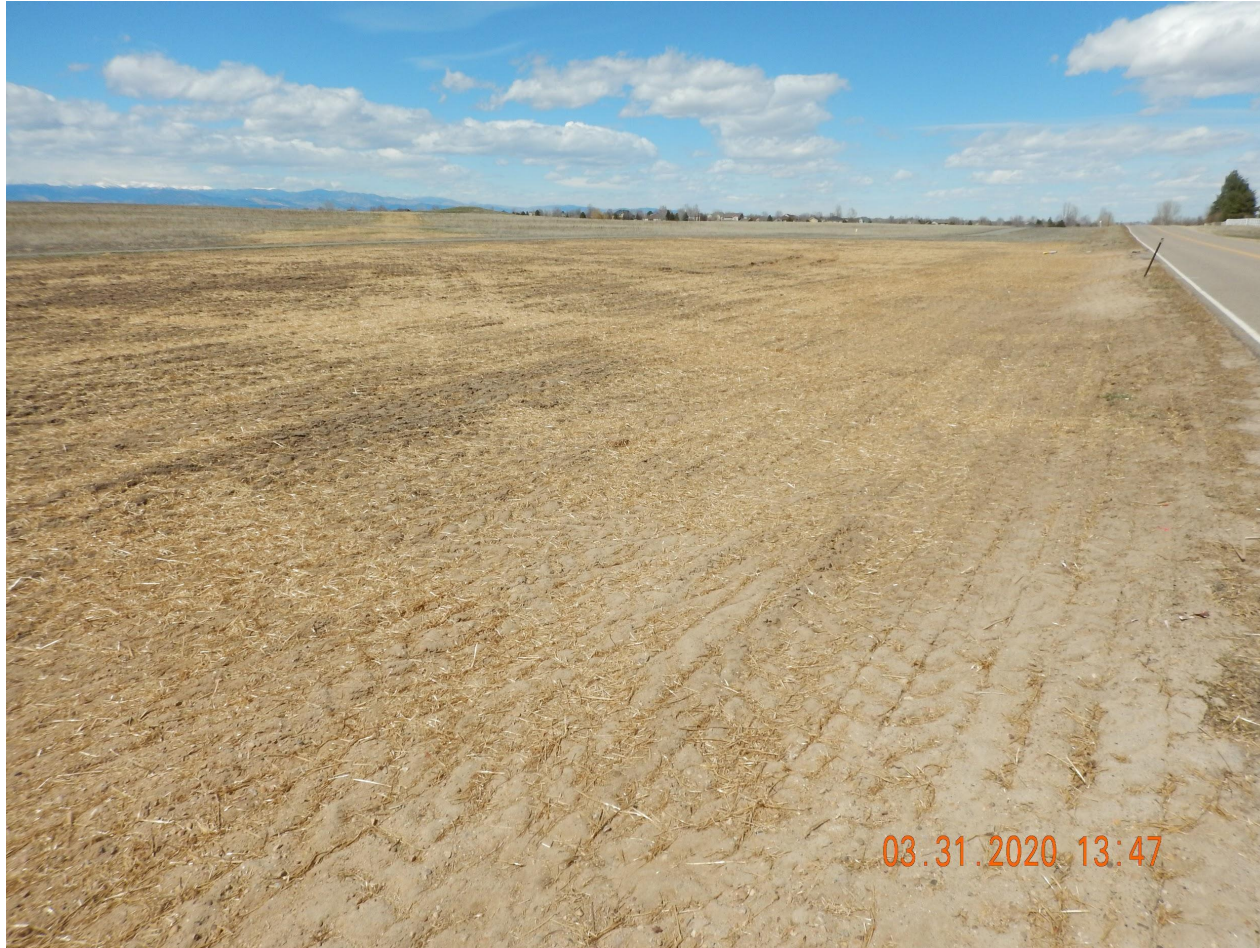
Photo 7. Photo taken from the offsite tank battery location, facing North. Photo illustrates Operator has removed all equipment from the associated offsite tank battery and has performed final reclamation activities with the evidence of drill rows and straw crimped mulch.
