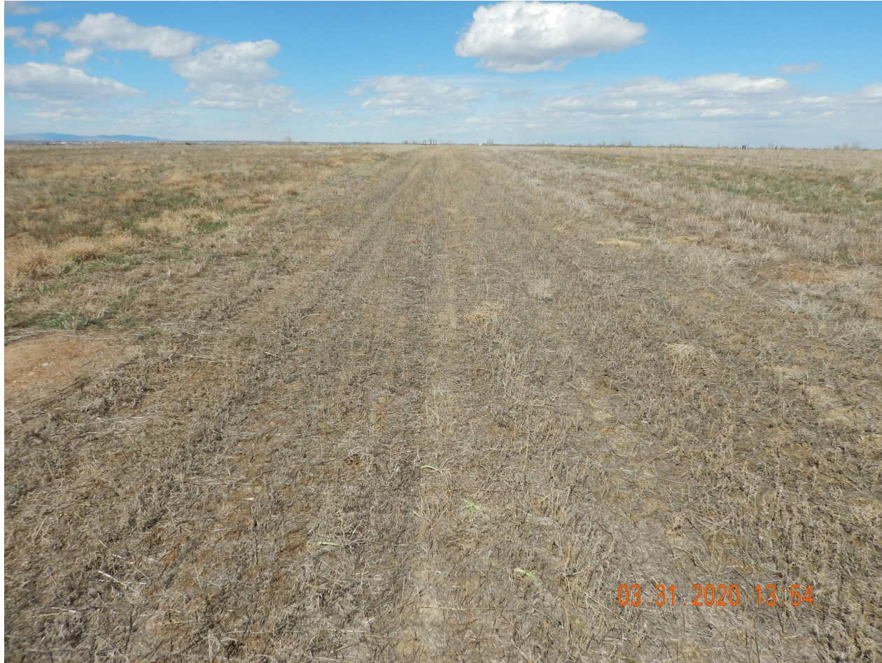
Photo 1. Photo taken from a portion of the well location access road, facing North. Photo illustrates the Operator has performed final reclamation activities but vegetation has not met Rule 1004 standards.
