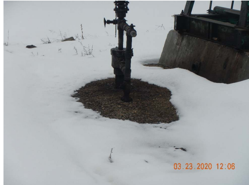
Photo 3. Close-up of wellhead soil staining.
