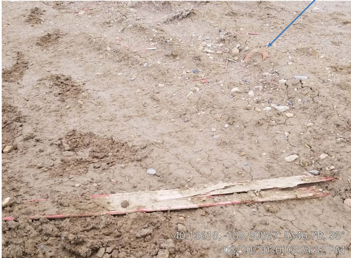
Photo 2. Fallen deadman in SW corner of location.
