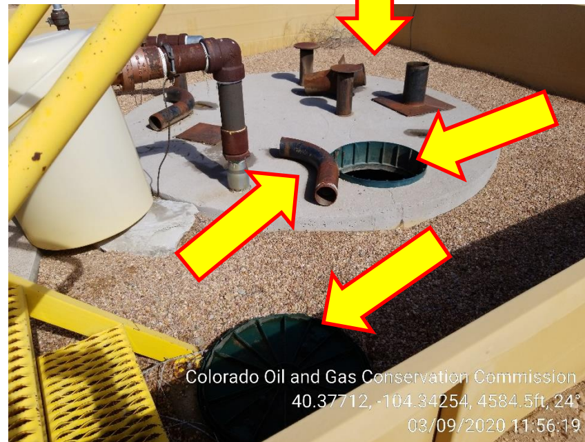
Photo 4 – Unused Pipe fittings at Maintenance Tank. Please replace Cover on Tank
