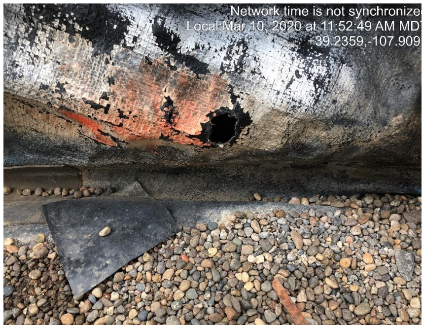
Photo #0734 Multiple holes through out tank containment liner.
