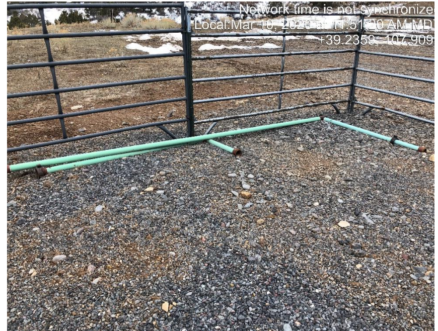
Photo #0733 Unused 2" piping by separators.
