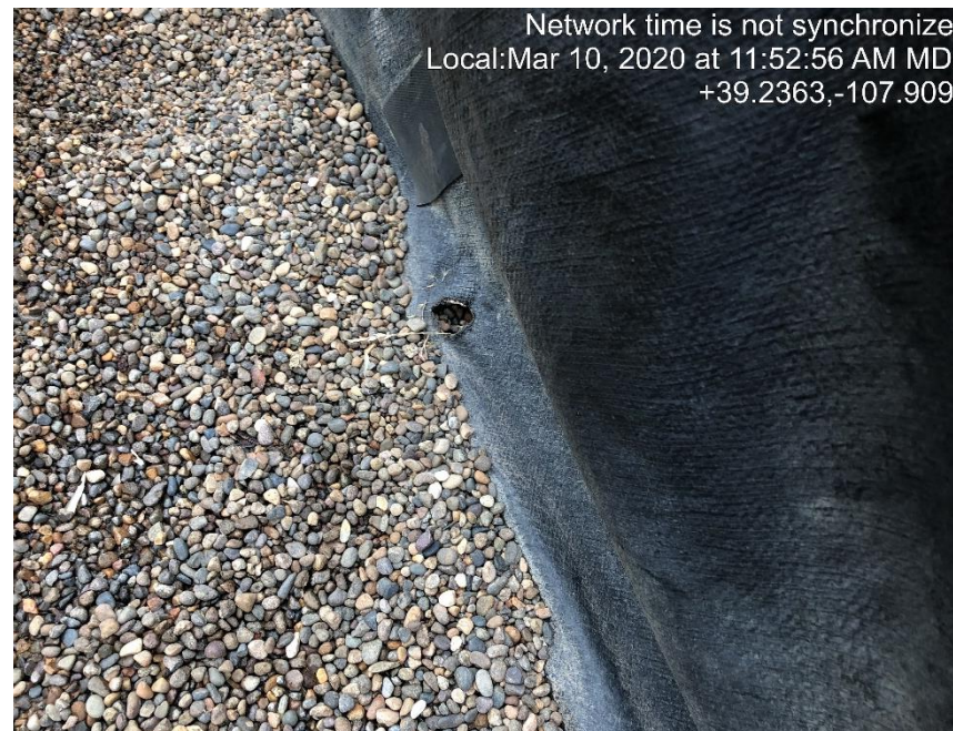
Photo #0735 Multiple holes through out tank containment liner.
