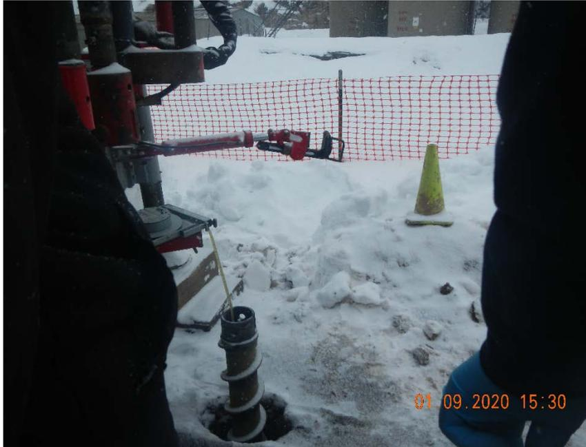
Photo #3 monitoring well install on west side of old cuttings storage pit. Note: production tanks in background.
