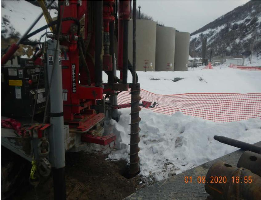
Photo #2 location of monitoring well. Note main tank battery in back. Construction fence is to prevent access to old soil storage area.
