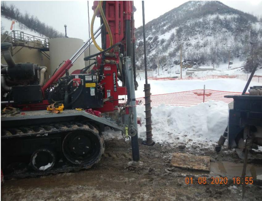
Photo #1 Drilling a groundwater observation well on the north side of old cuttings pit.
