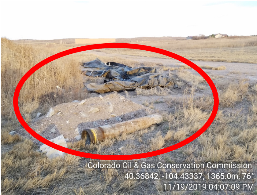
Photo #3 DOW 43-28 Wellsite Plugged & Abandoned | PA Junk & Trash Cut casing pipe, cement, plastic liner
