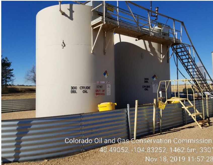
Photo 5: Tank Battery
