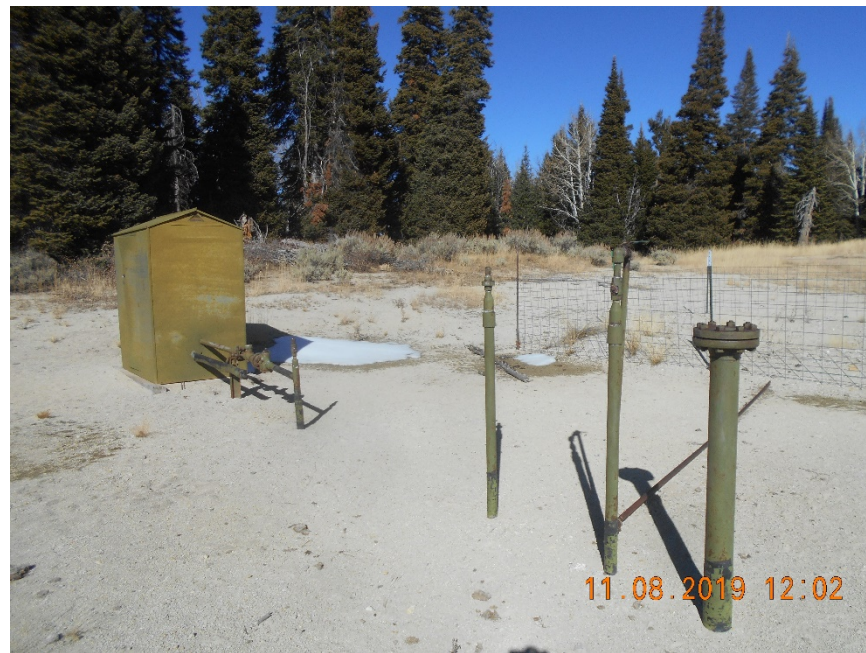
Meter housing. Flowline risers disconnected.
