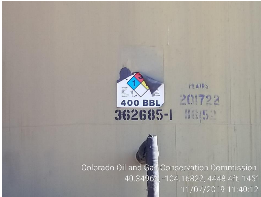
Photo 3 – Middle Tank – Content and NFPA Label
