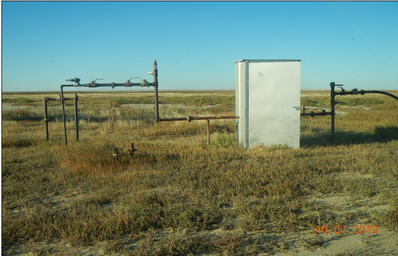
Photo 4. Pipe risers at the location have no LO/TO.
