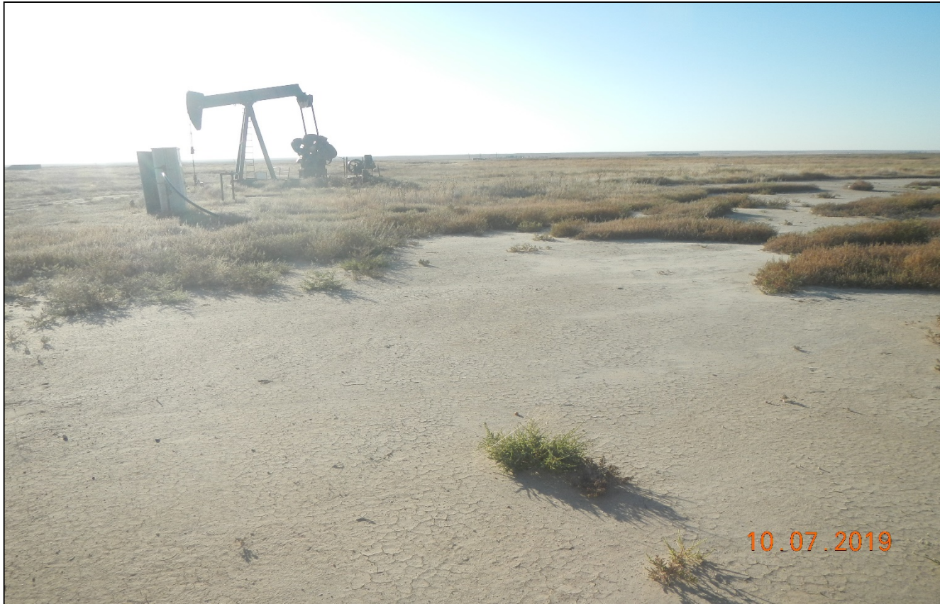
Photo 5. Facing west toward the wellhead. The area northeast of the well is bare of vegetation and appears to be a result of a spill.
