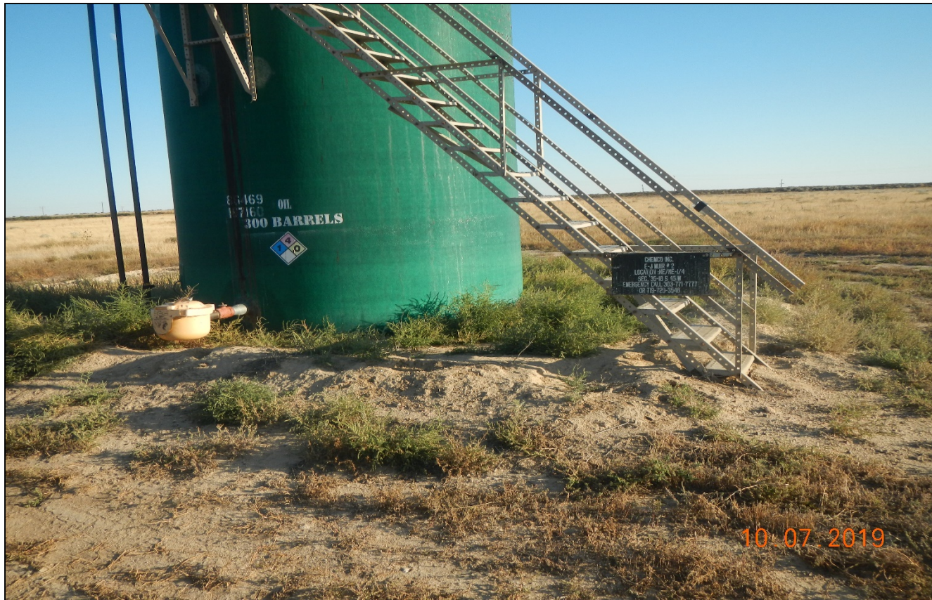
Photo 3. The berm around the tank is degraded and not sufficient to contain a spill.
