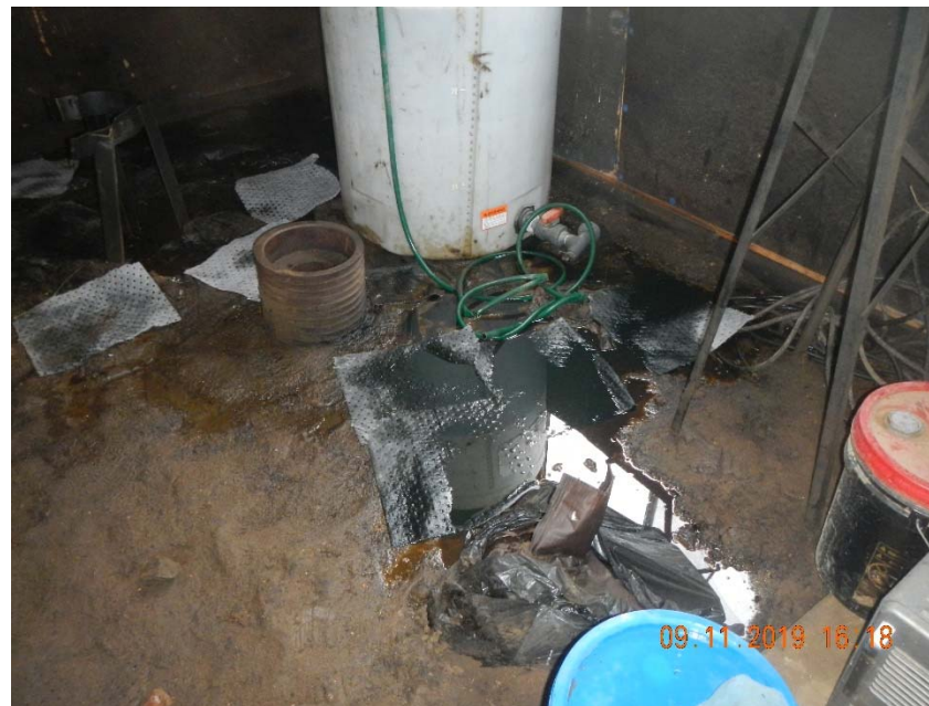
Photo 6. Free fluid and stained soil in pump building.
