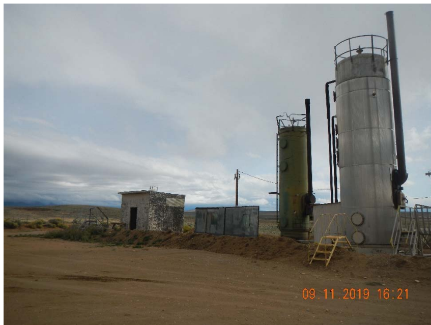
Photo 9. Berm does not appear compacted.
