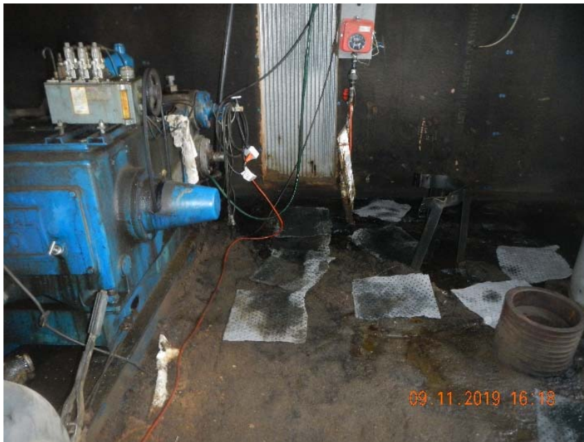
Photo 7. Free fluid and stained soil in pump building.
