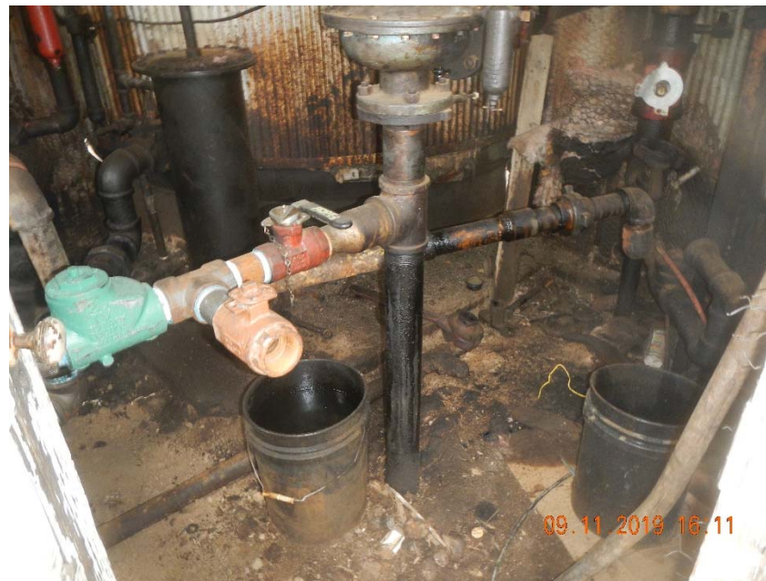
Photo 4. Free fluid and stained soil in separator building.
