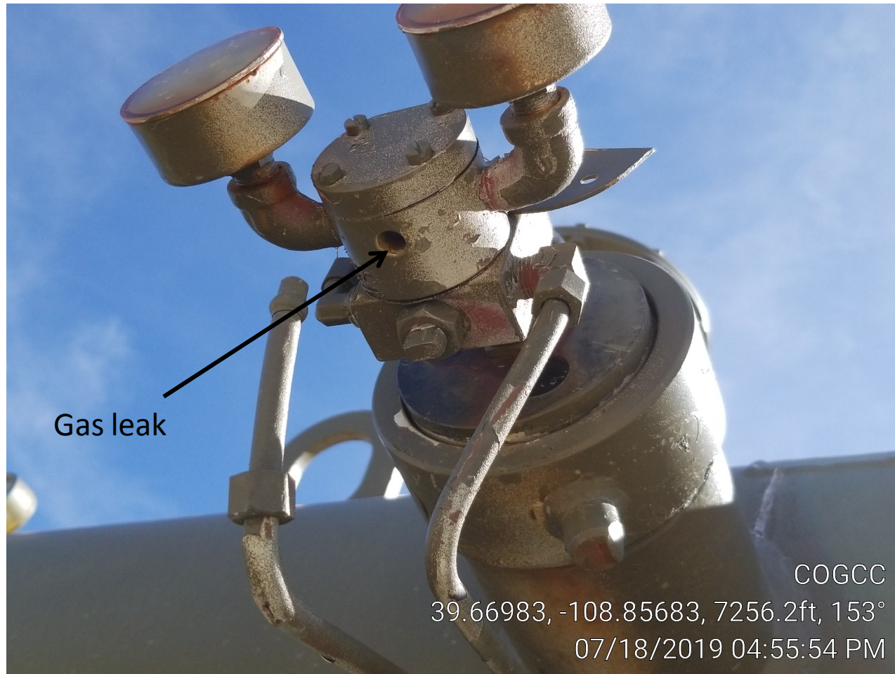
Photo 5. Gas leak at separator on 7-18-2019.
