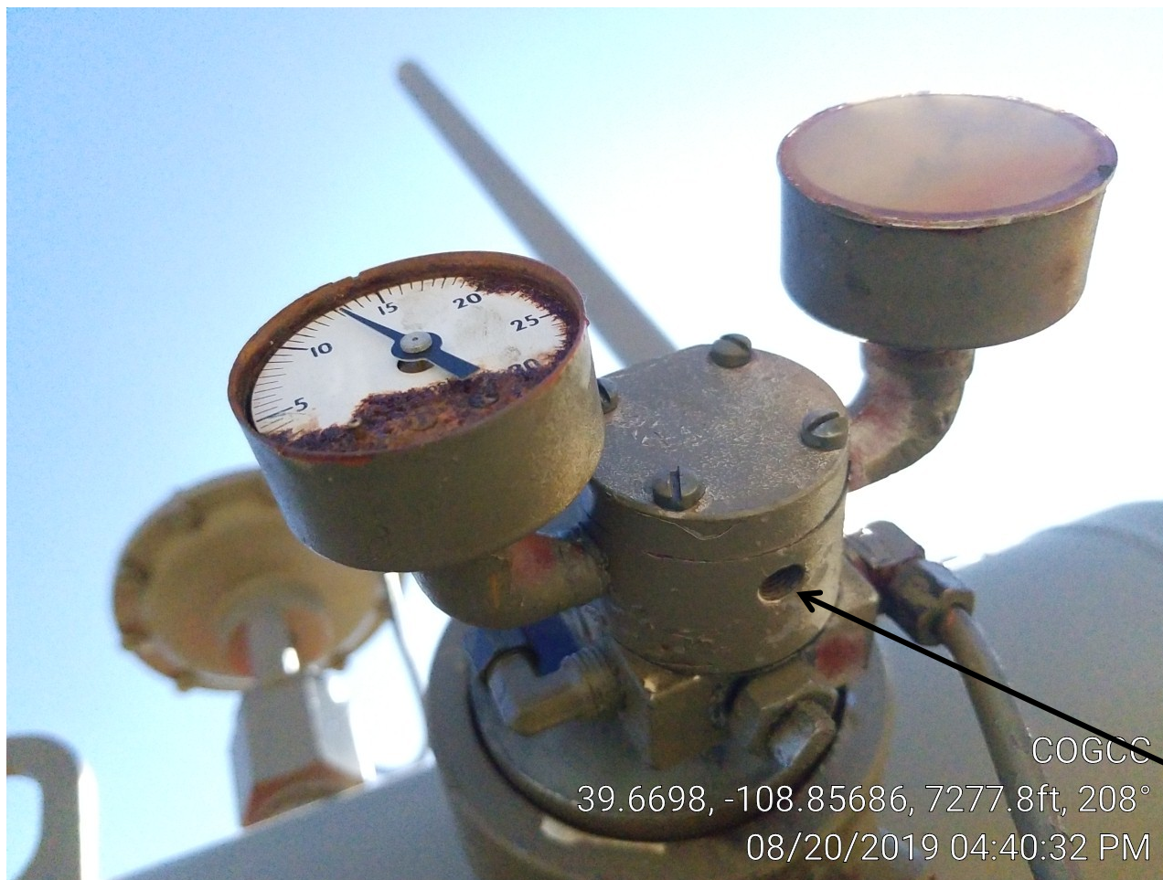
Photo 4. Separator gas leak.
