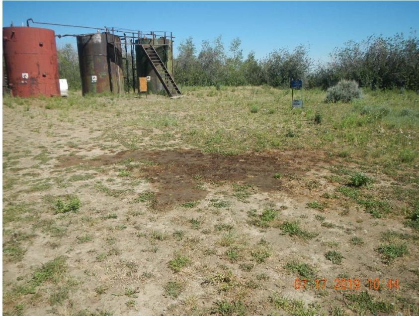
Photo 3. Stained soil on location between wellhead and tank battery.
