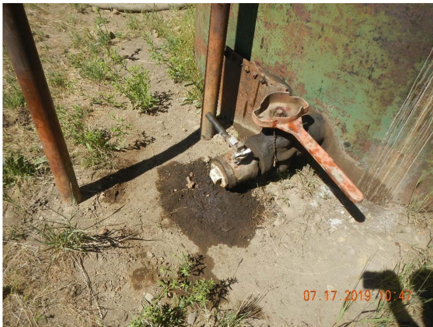
Photo 11. Stained soil at tank loadout valve.
