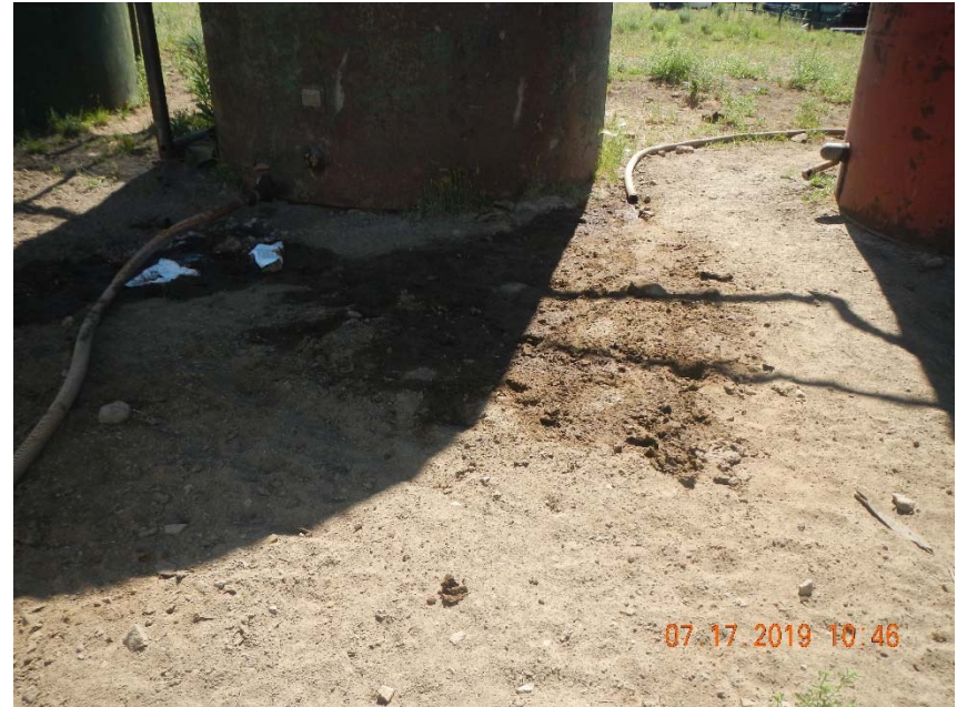
Photo 6. Stained soil and debris in tank battery.
