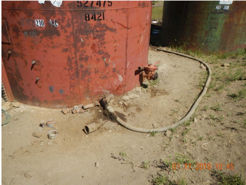
Photo 5. Stained soil at tank loadout valve.
