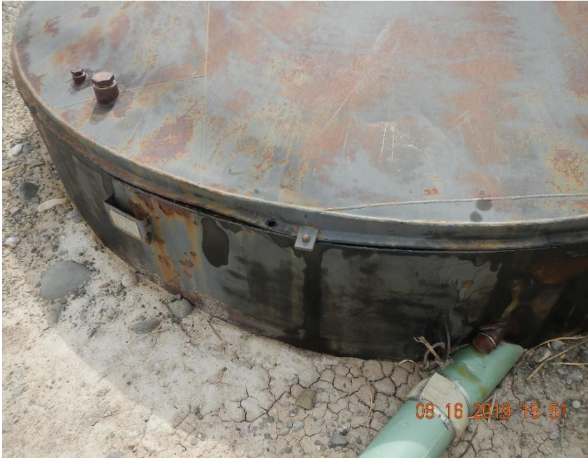
Top seam of PBV appears to be damaged. PBV is rusty and requires painting and labeling per Rule 210.d.
