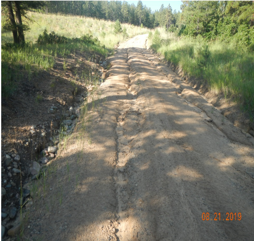
Photo 2. There is erosion issues along the access road to the location.
