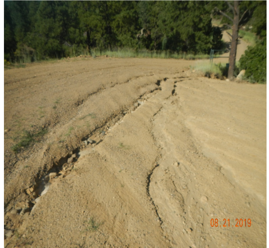
Photo 1. There is signs of erosion along the main road near the Led 31-21 location.
