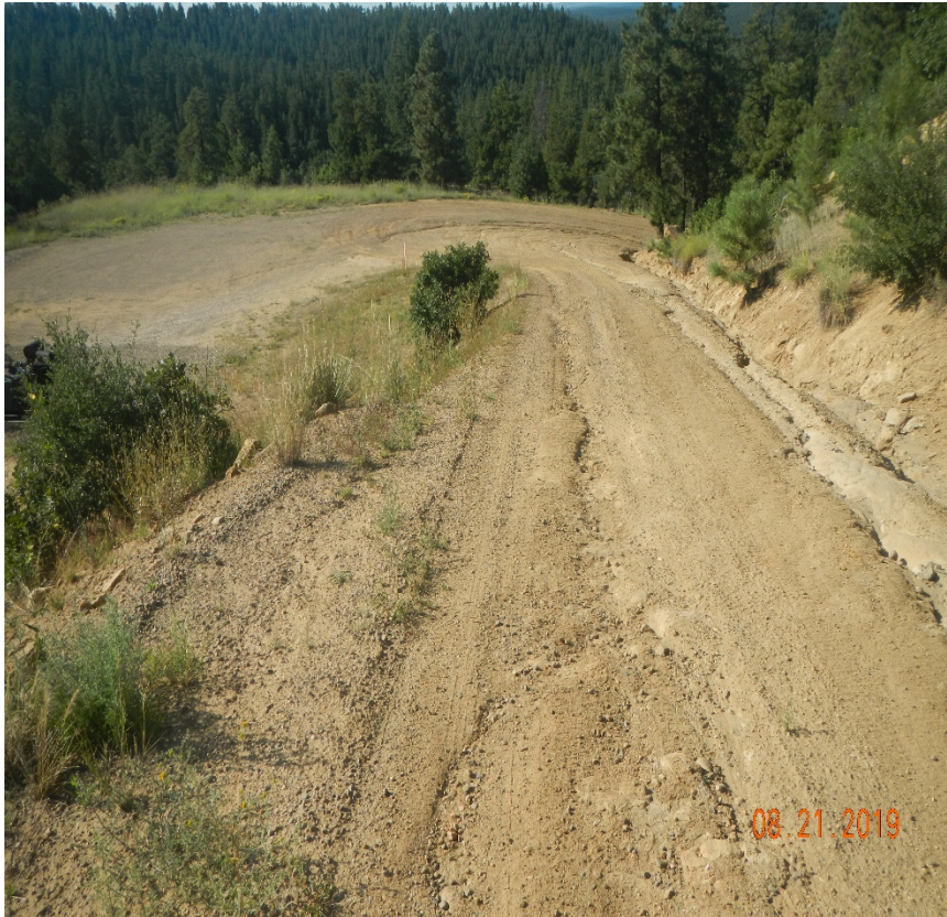
Photo 1. There is signs of erosion along the main road near the Led 31-21 location.
