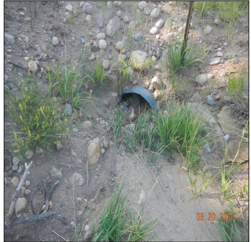
Photo 4. The erosion channel leads to the culvert which is partially filled in..
