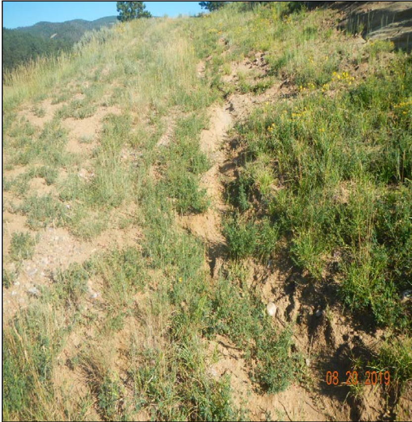
Photo 3. There is an erosion channel along the road.
