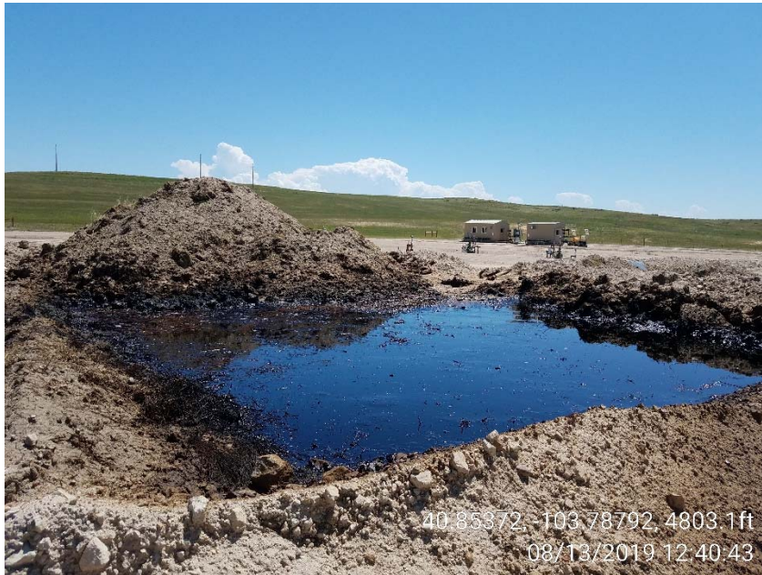
Photo 1 – Stockpile 1 of 2 of impacted material from Horsetail 7CPB spills in bermed lined containment. Free oil present.
