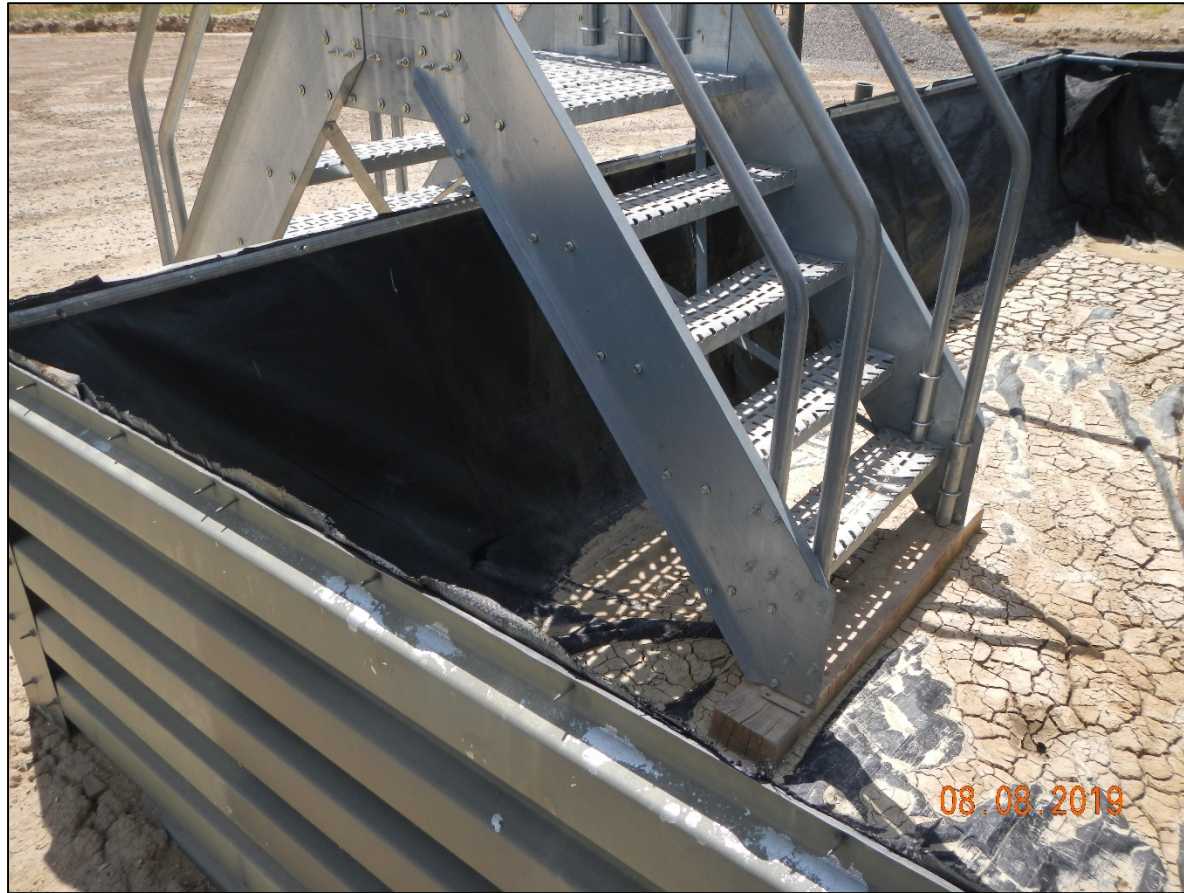
Photo # 10 hole in tank containment liner by steps
