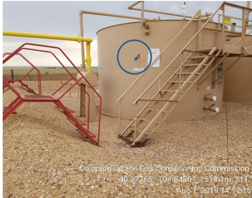
Photo 3: NFPA placard needs to be replaced
