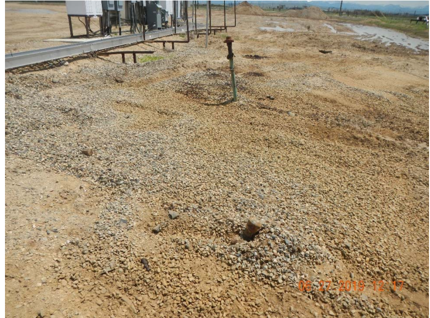
Photo 8. 2 risers not LOTO or marked for abandonment.
