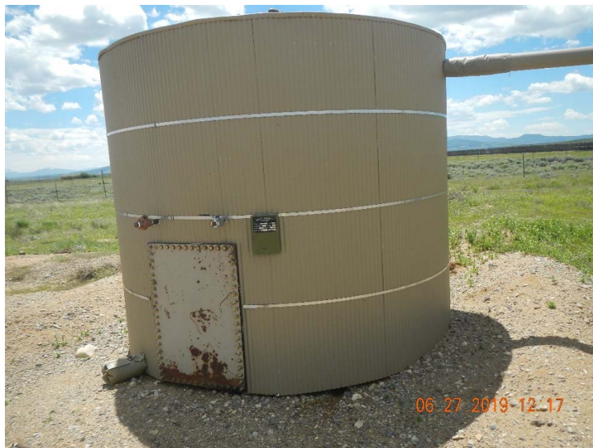
Photo 1. Unlabeled tank with no apparent berm or liner.
