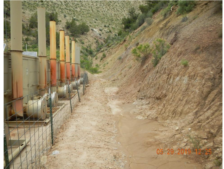
Sediment build up in ditch behind separators.
