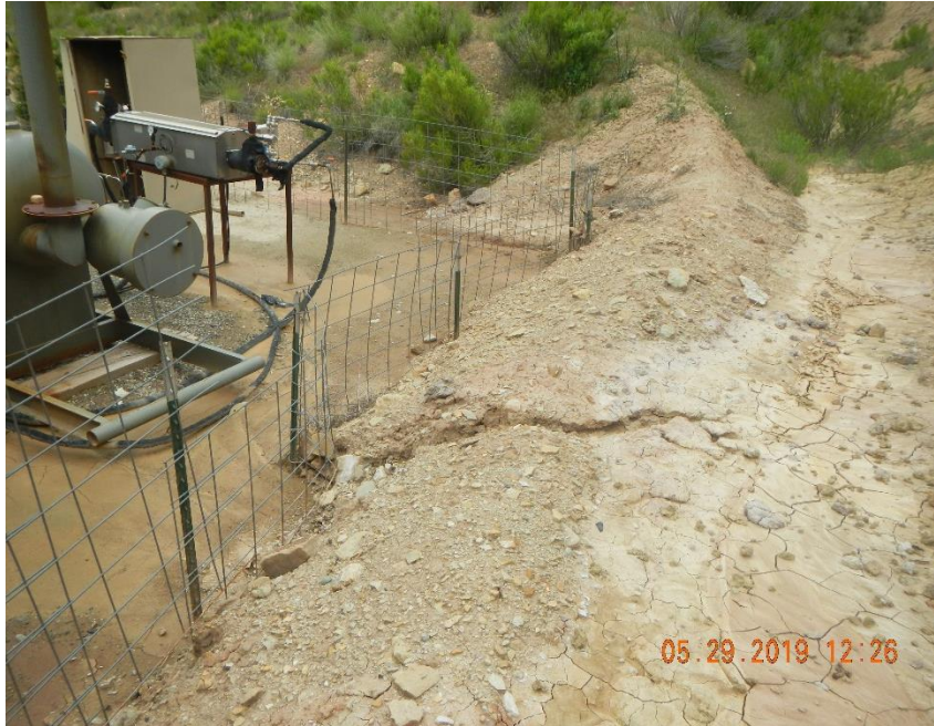
Breach in ditch wall.
