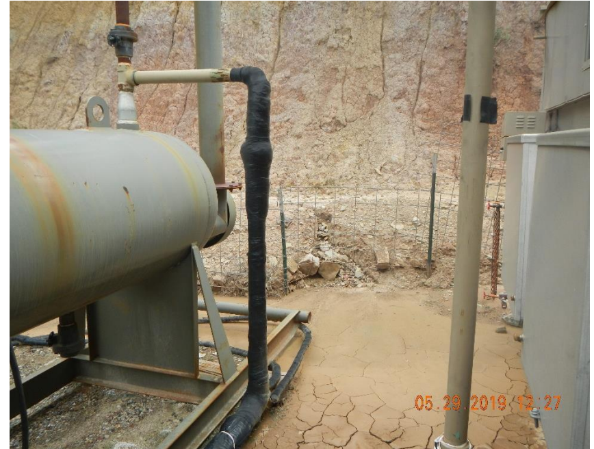
Breach running into separators.
