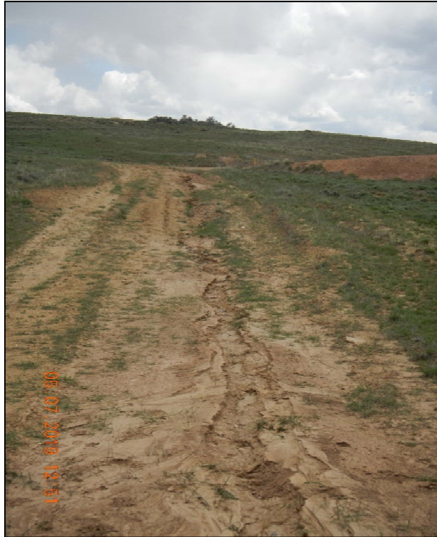
Photo 2. Sediment moving off location onto access road.
