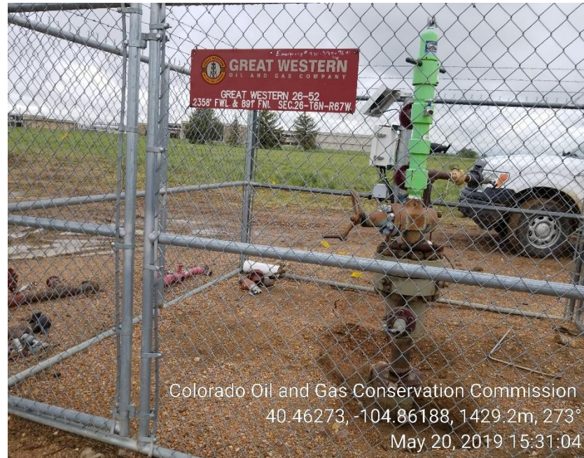
Photo 1: Wellhead; unused equipment, Emergency Contact # NOT legible.
