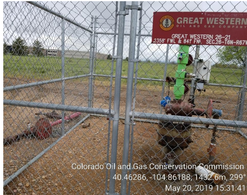
Photo 1: Wellhead; unused equipment, Emergency Contact # NOT legible.
