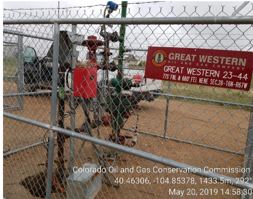
Photo 1: Wellhead; unused equipment, No Emergency Contact #.
