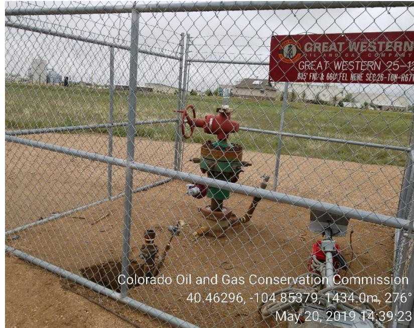
Photo 1: Wellhead; unused equipment, No Emergency Contact #.
