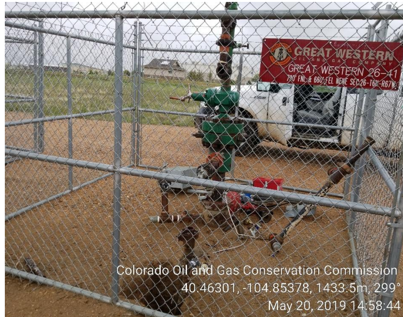
Photo 1: Wellhead; unused equipment, No Emergency Contact #.
