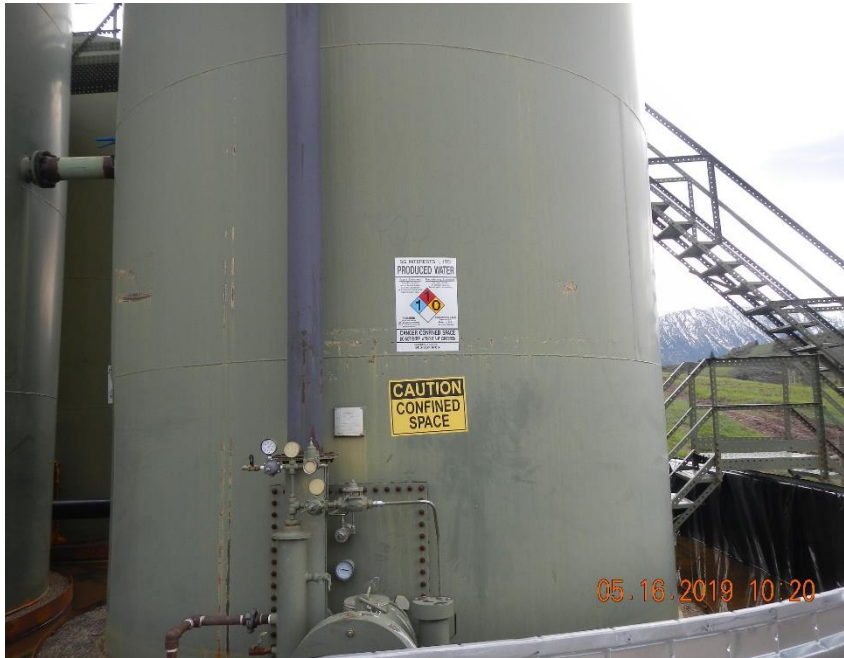
ASTs are no longer labeled with capacity.
