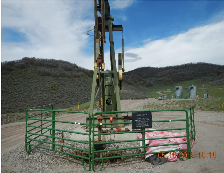
Federal 11-90-24 #1 well head and pump jack.
