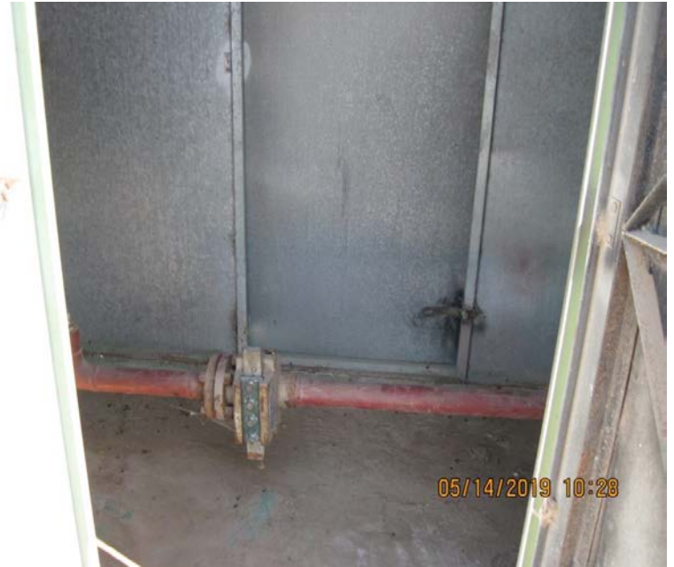
2. Gas meter has been removed
