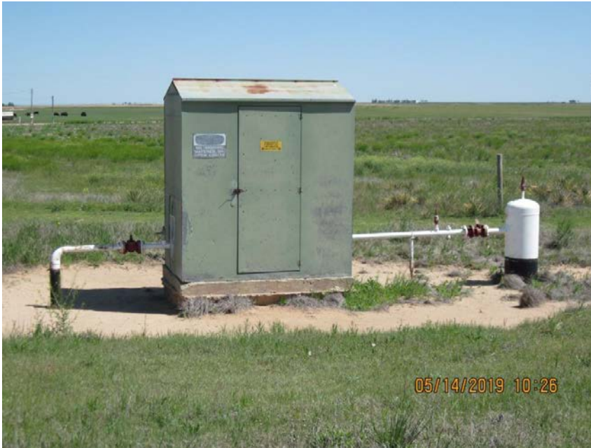
1. Meter run and Vertical gas separator
