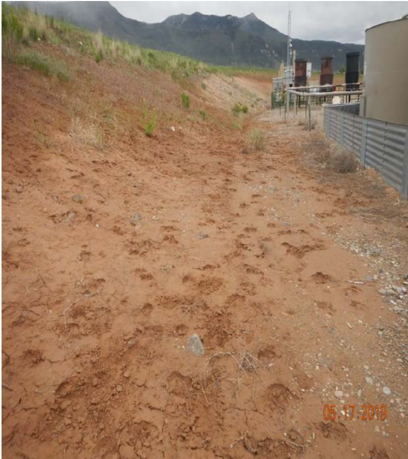
Photo#8: Cut slope needs to be stabilized.
