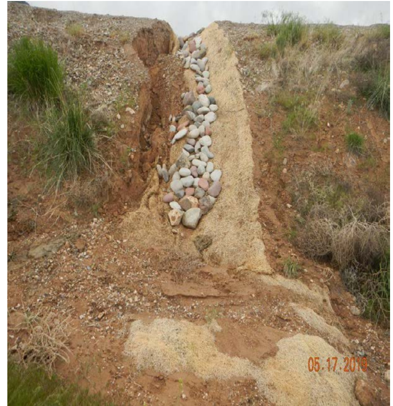
Photo#7: Washed out BMP at North end of site.
