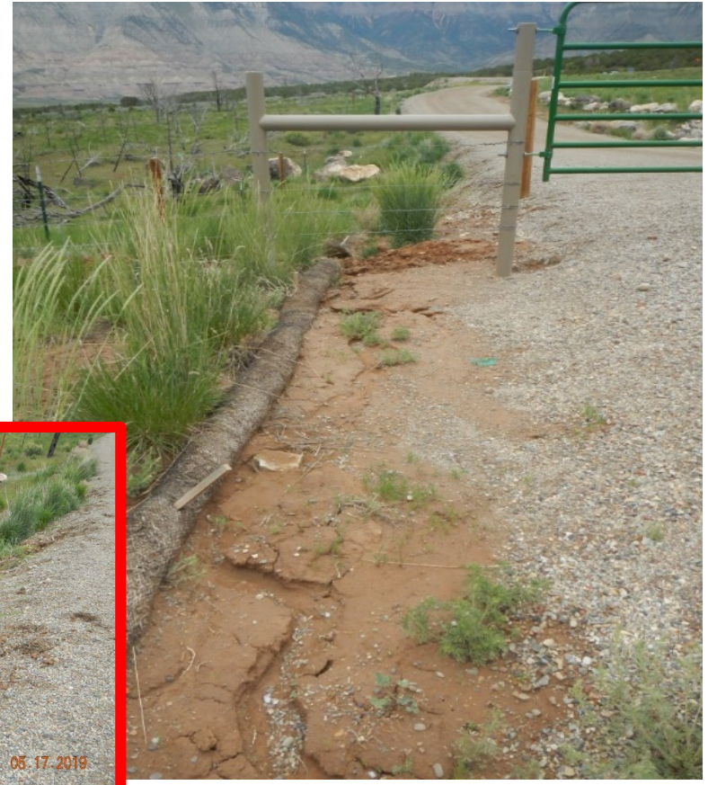
Photo#5: BMPs on access road need maintenance
