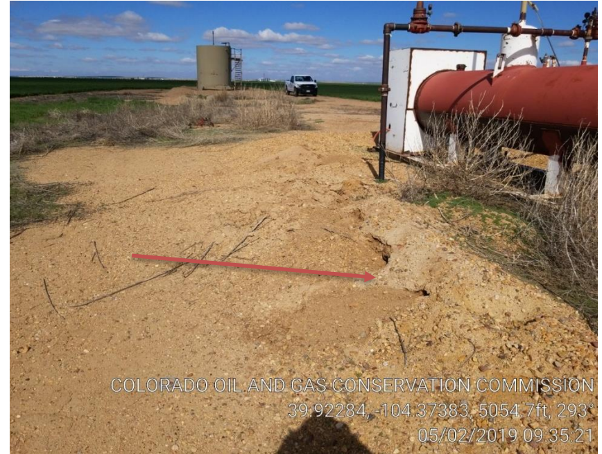
Pic 6 separator berm appears to have burrowed through by animals.
