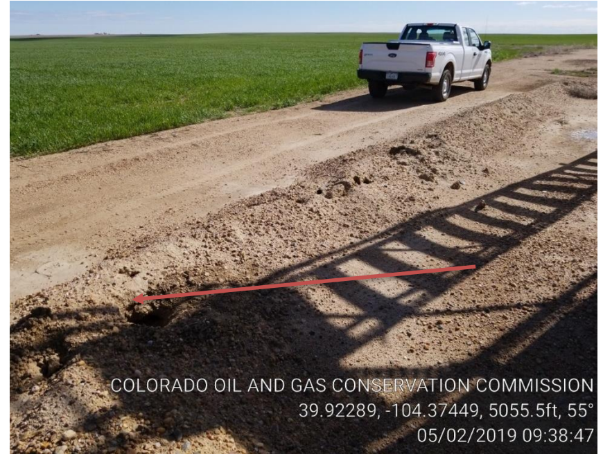
Pic 11 berm appears to have been burrowed through by animals
