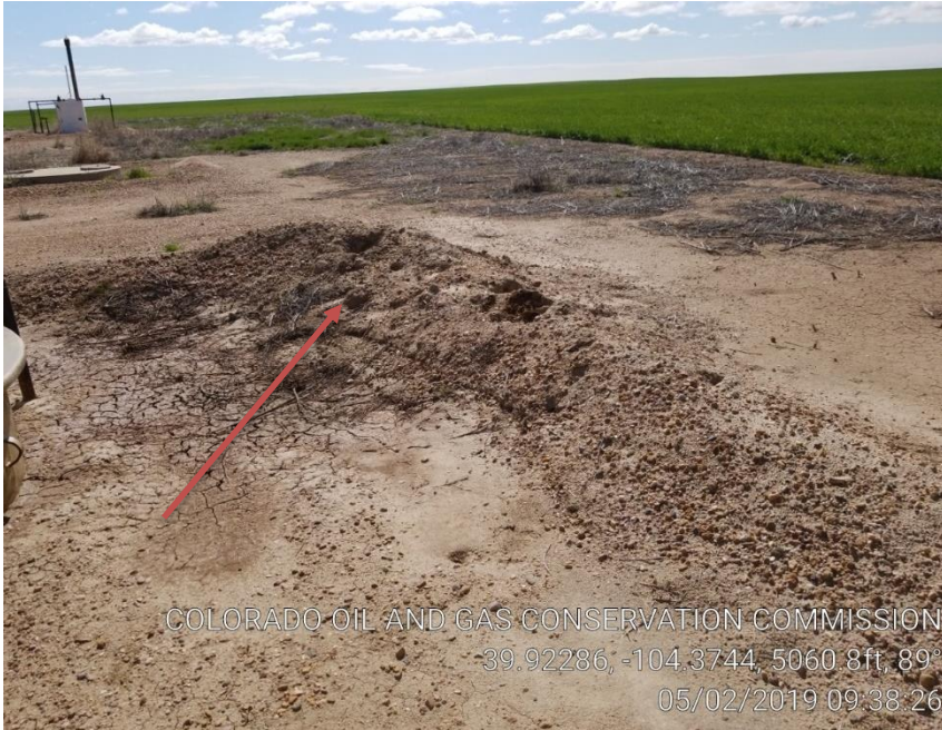
Pic 11 berm appears to have been burrowed through by animals.
