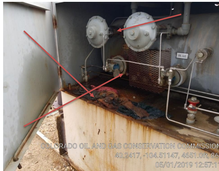
Pic 4 possible leak
