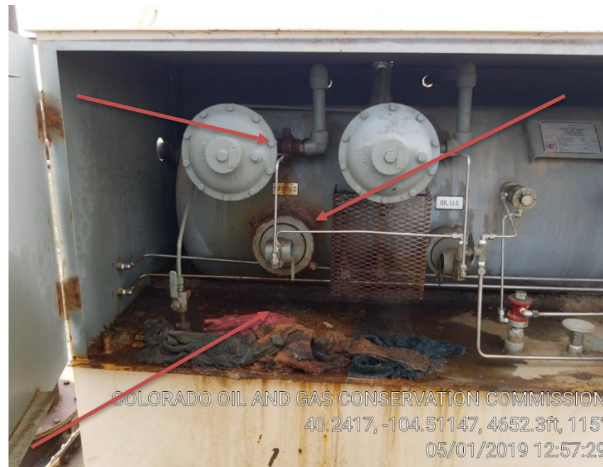
Pic 6 possible leak
