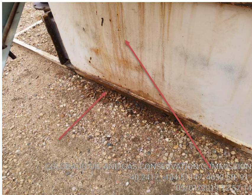
Pic 5 possible leak stained soil.
