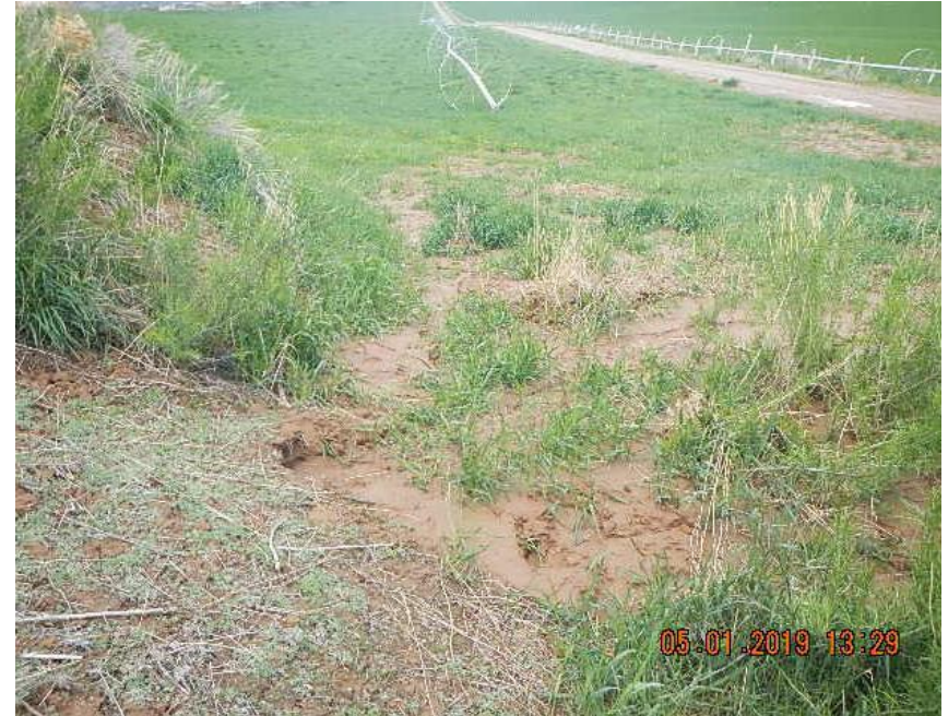
Run off and sediment movement at fill slope
