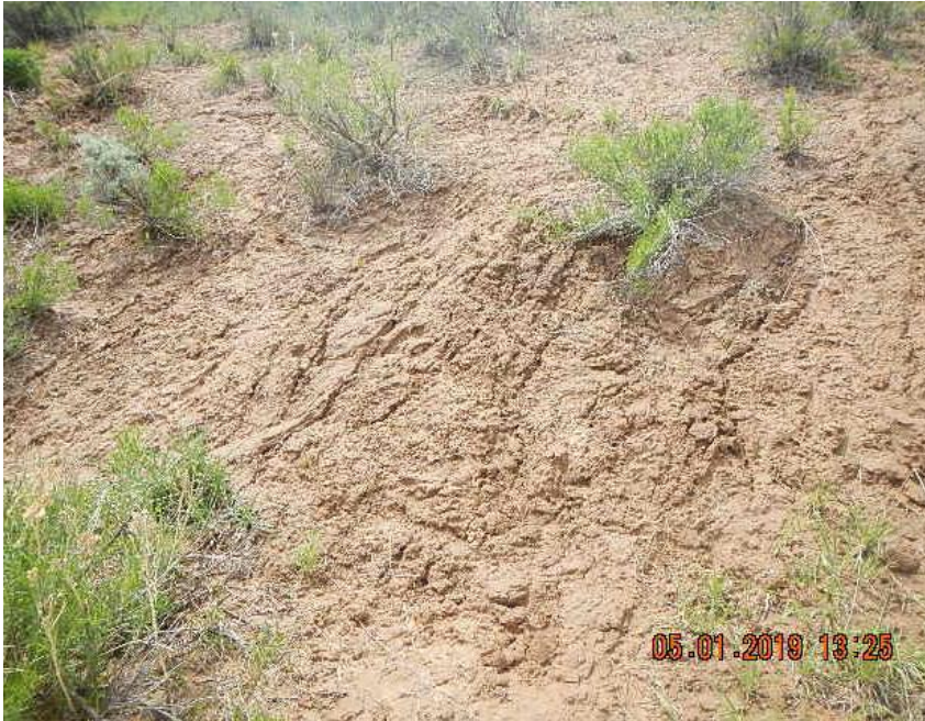
Run on and sediment moving onto pad surface
