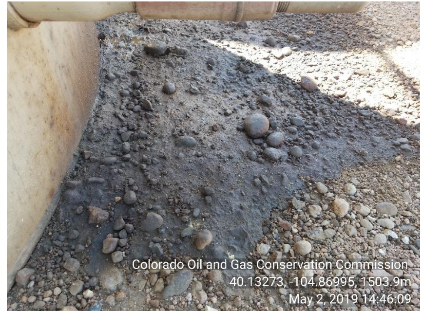
Photo 6 Ground saturated from what appears to a leak at bottom of produced water tank.
