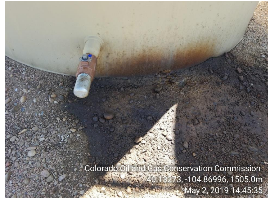
Photo 4 Ground saturated from what appears to be a leak at bottom of produced water tank. Mechanical issue: leak on tank.
