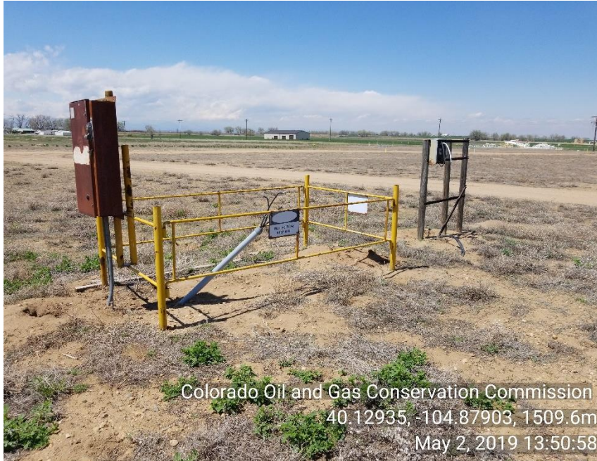
Photo 1 Unused equipment: bare electric wires, electric panel's and guard.
