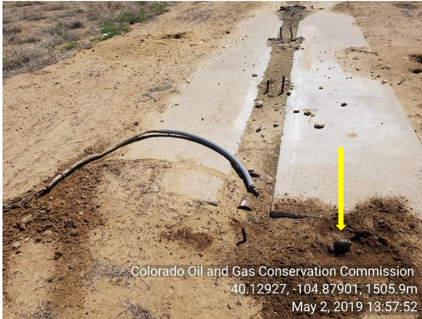
Photo 5 Unmarked unused and not LOTO riser. Trash electric line, spark plugs
