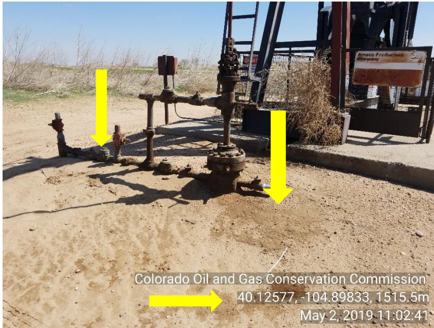
Photo 5 Stained soil around WH
