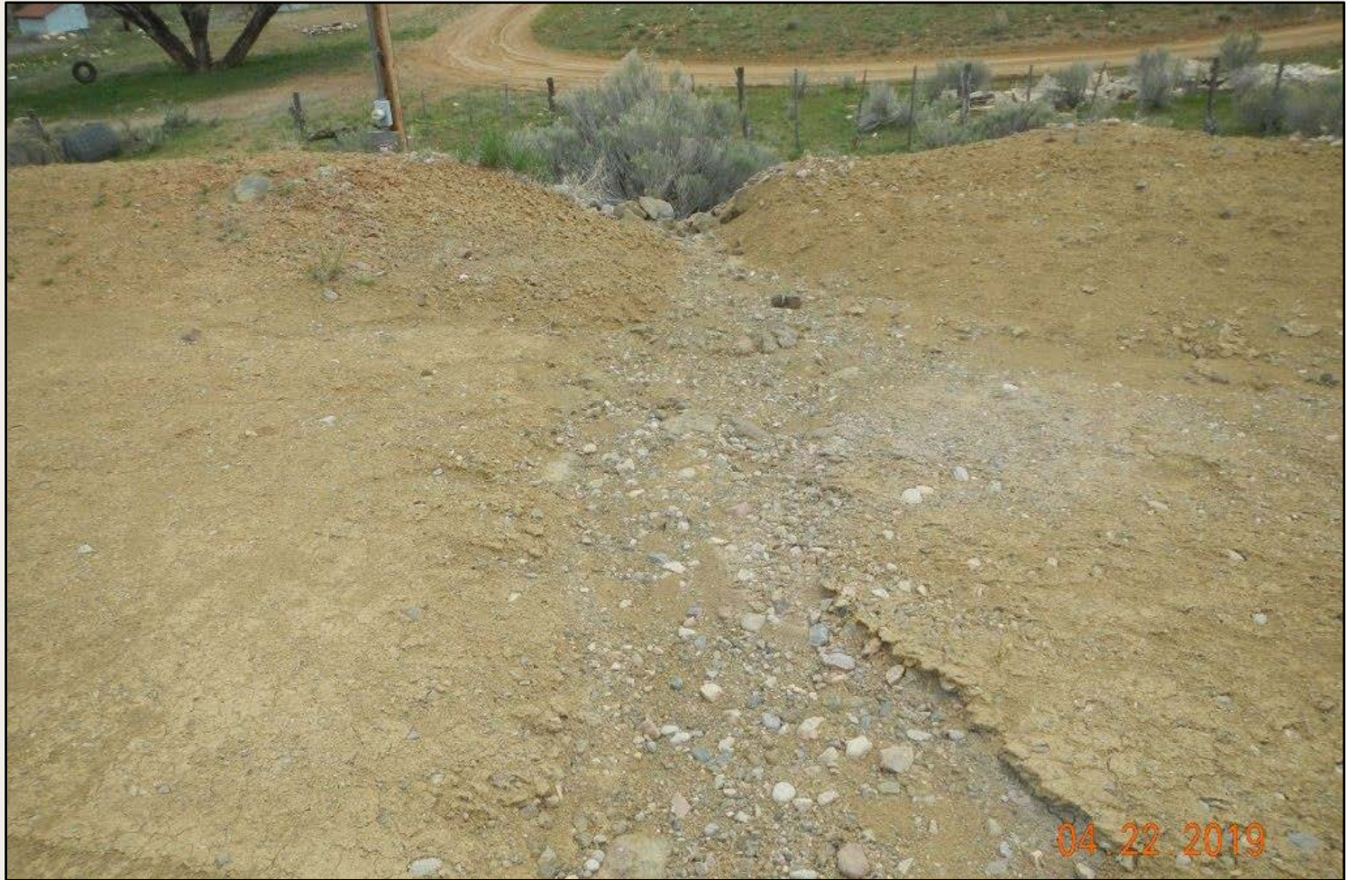
Photo 3. View of erosional scouring in the southern project area where concentrated stormwater flows off of the well pad.
