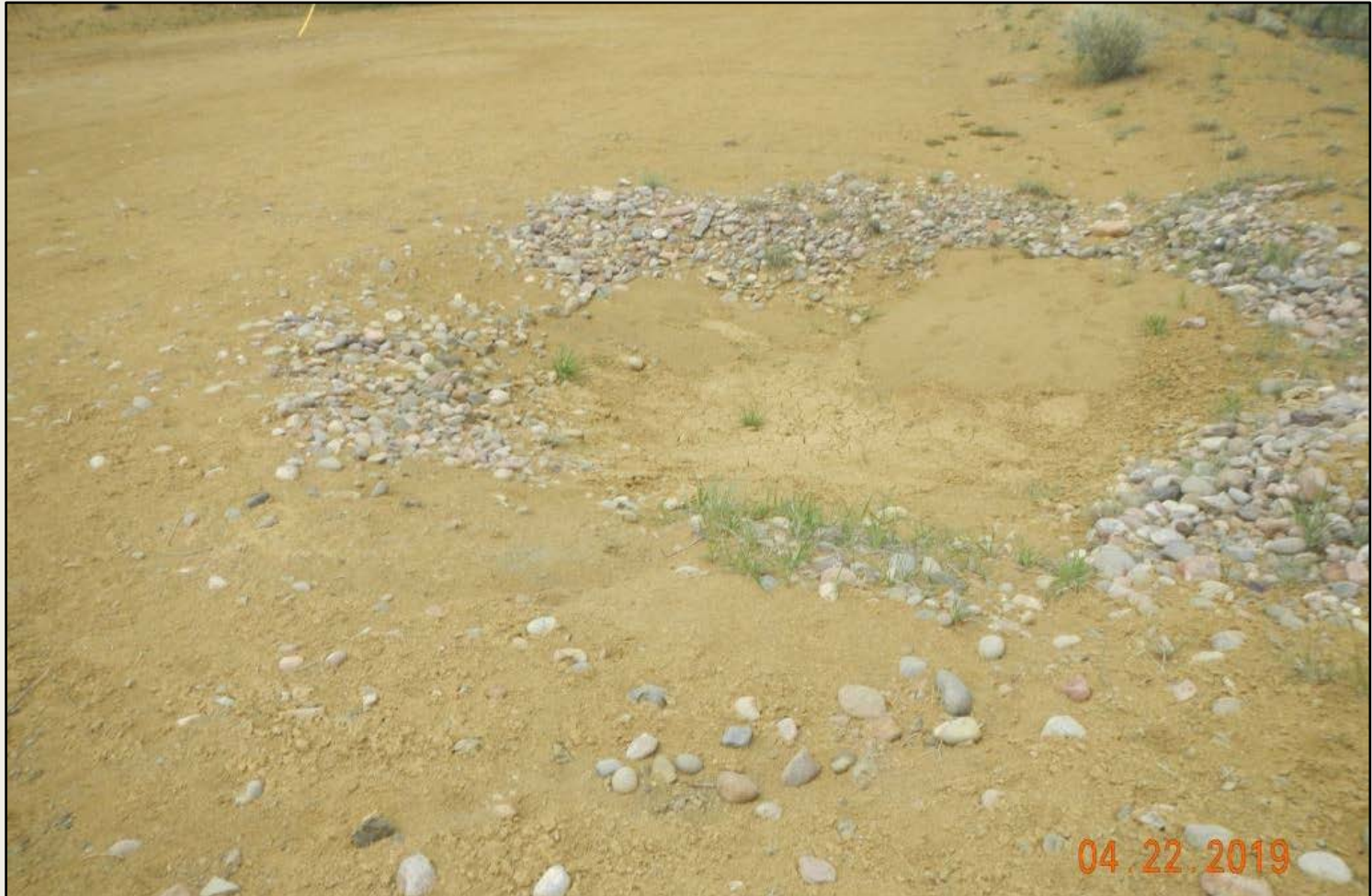
Photo 2. View of silt trap in the eastern project area that is full of sediment.
