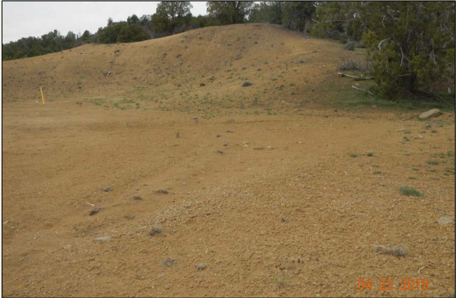
Photo 4. View of the northwestern cut-slope that is not properly stabilized.
