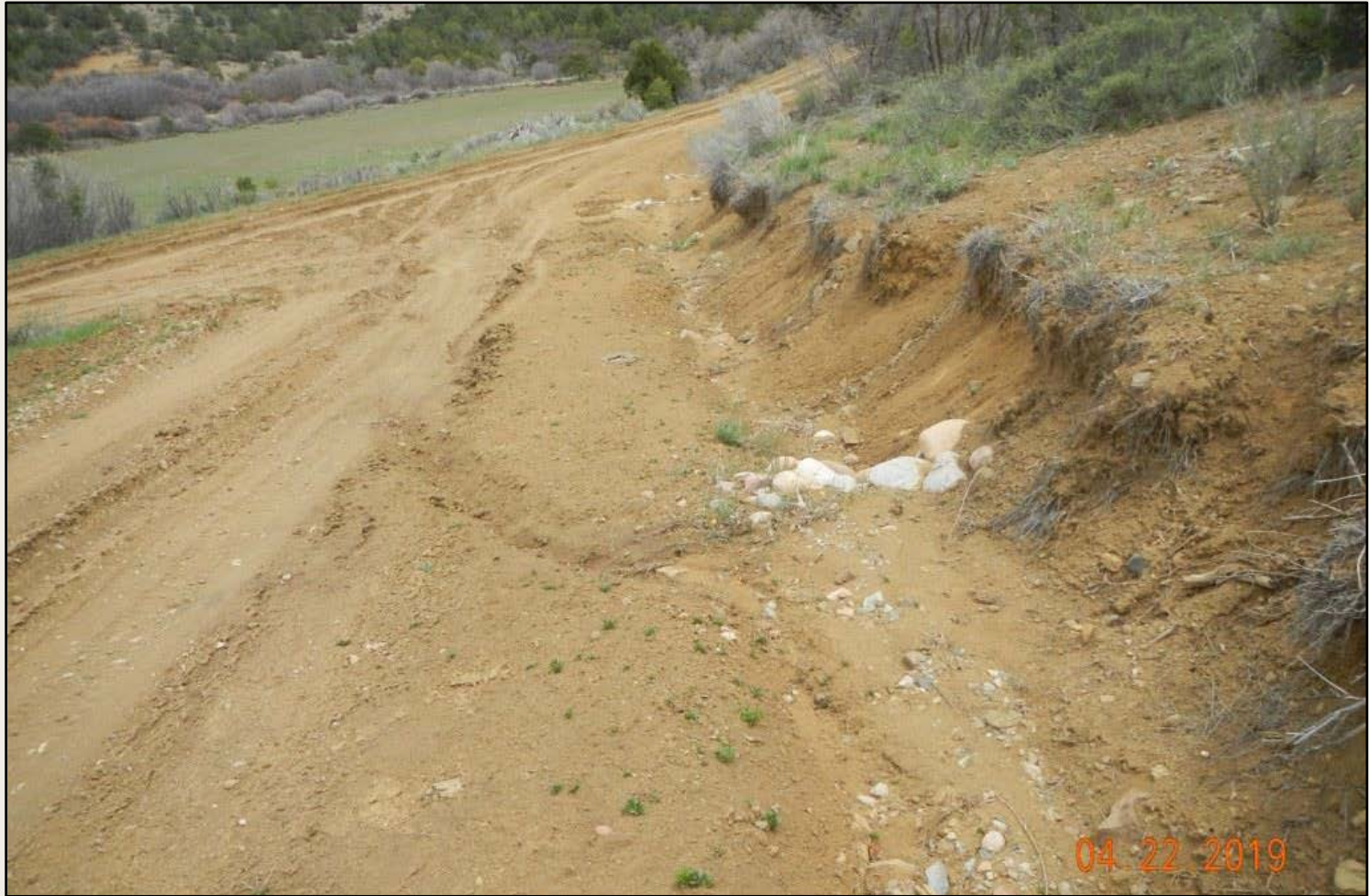
Photo 3. View of erosion, sedimentation, and insufficient stormwater controls along the access road.
