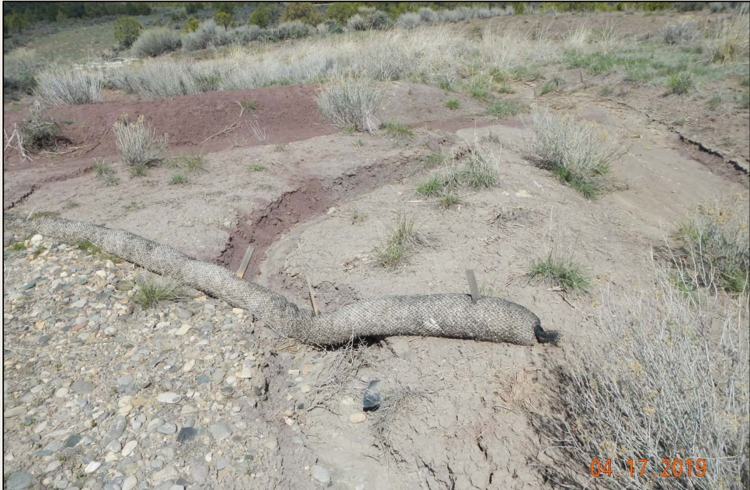
Photo 5. View of wattle in the northern project area that is not functioning.
