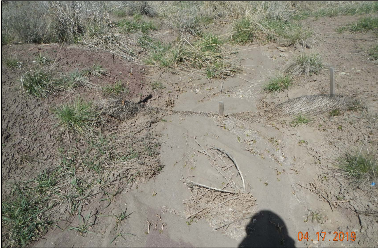
Photo 4. View of wattle in the northern project area that is full of sediment.
