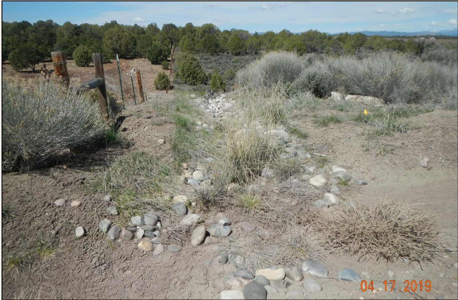
Photo 6. View of cobble run-down within the western project area that needs maintenance due to sediment accumulation.
