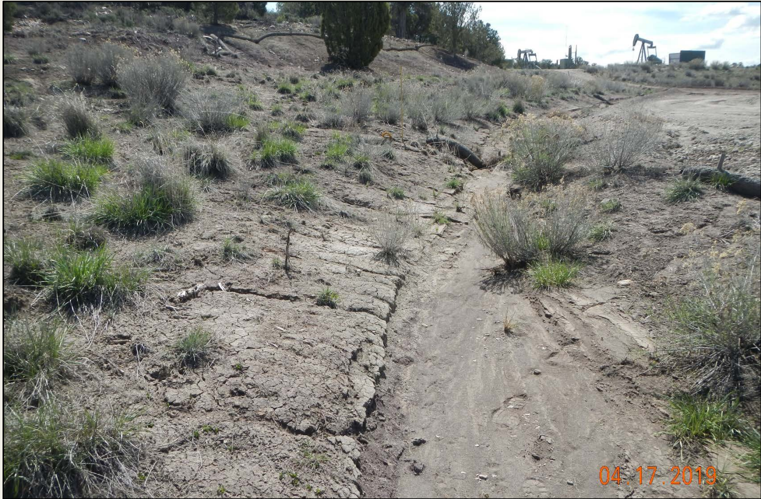
Photo 2. View of eastern diversion ditch that is full of sediment and eroding. Additional stabilization is needed here.
