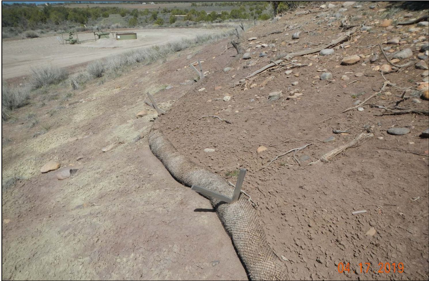
Photo 1. View of wattles in the eastern project area that are full of sediment.
