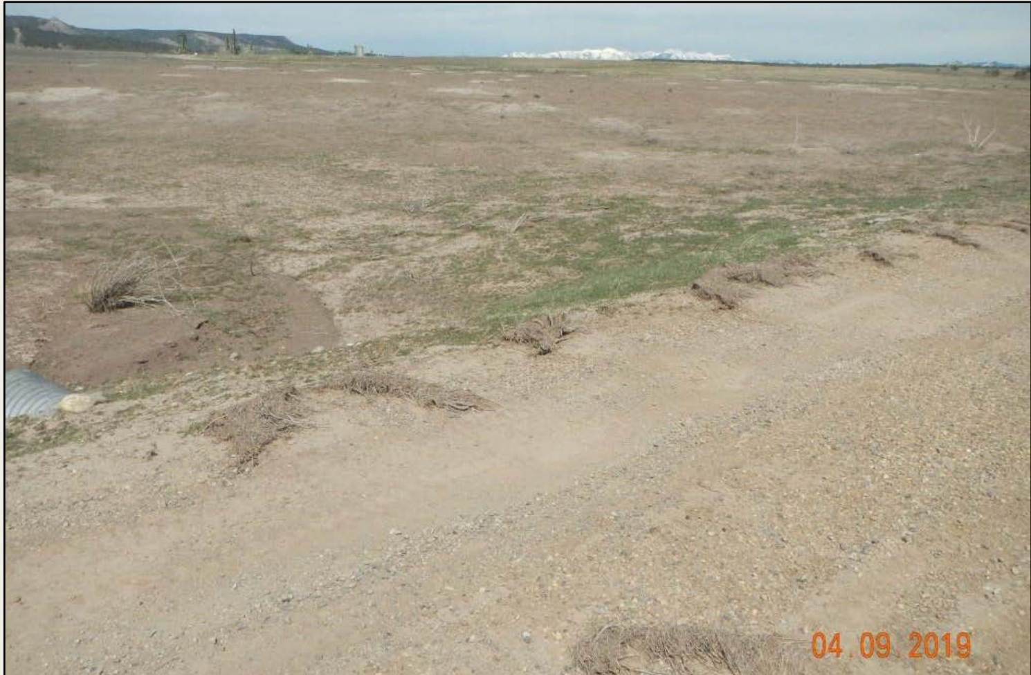
Photo 4. View of area along access road where it appears stormwater flows recently crossed over the road (facing upstream), indicating that culvert is not adequately sized/designed.
