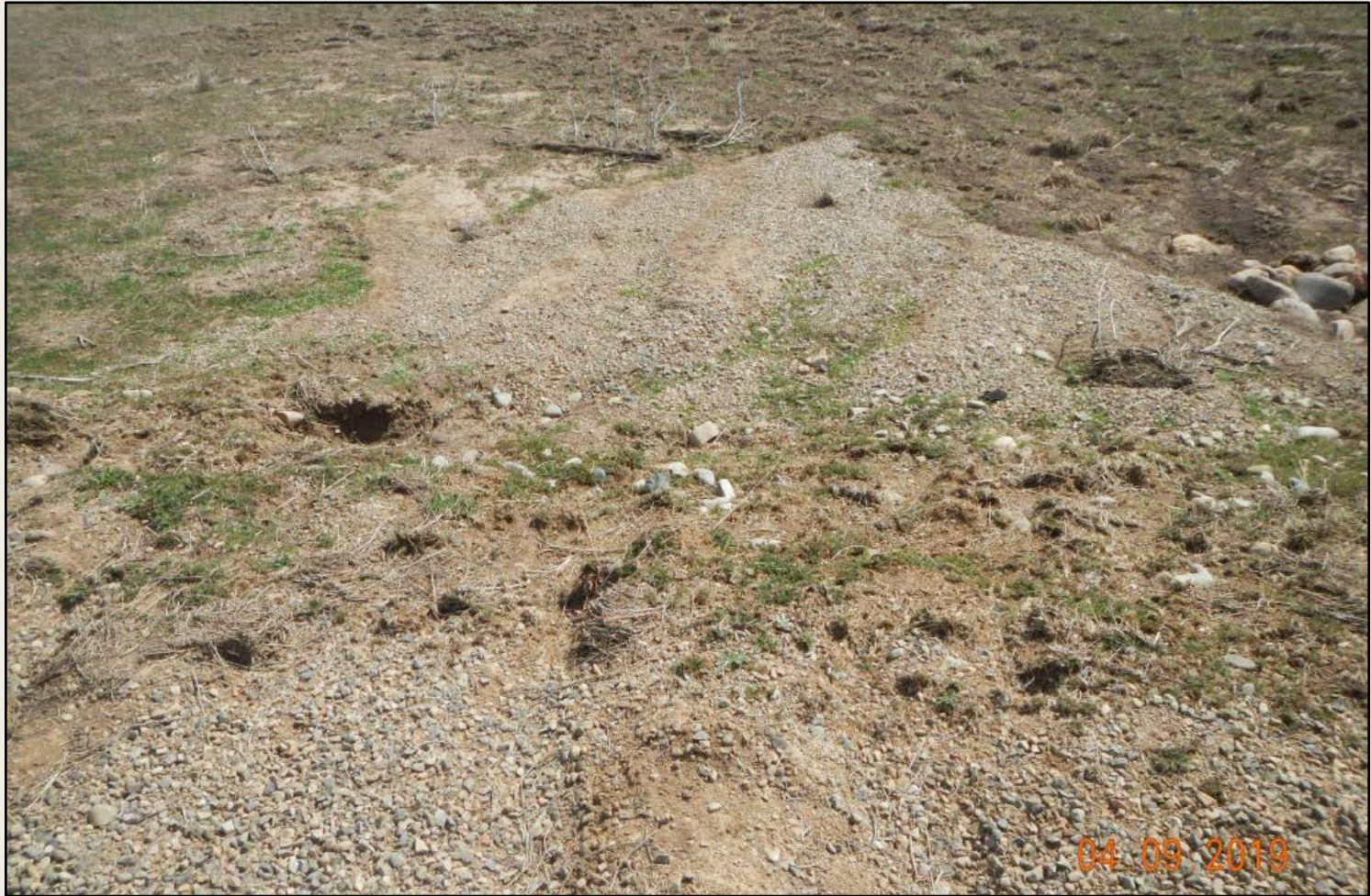
Photo 5. View of area downstream from Photo 4, where stormwater flows recently crossed over the road, depositing sediment from the road.
