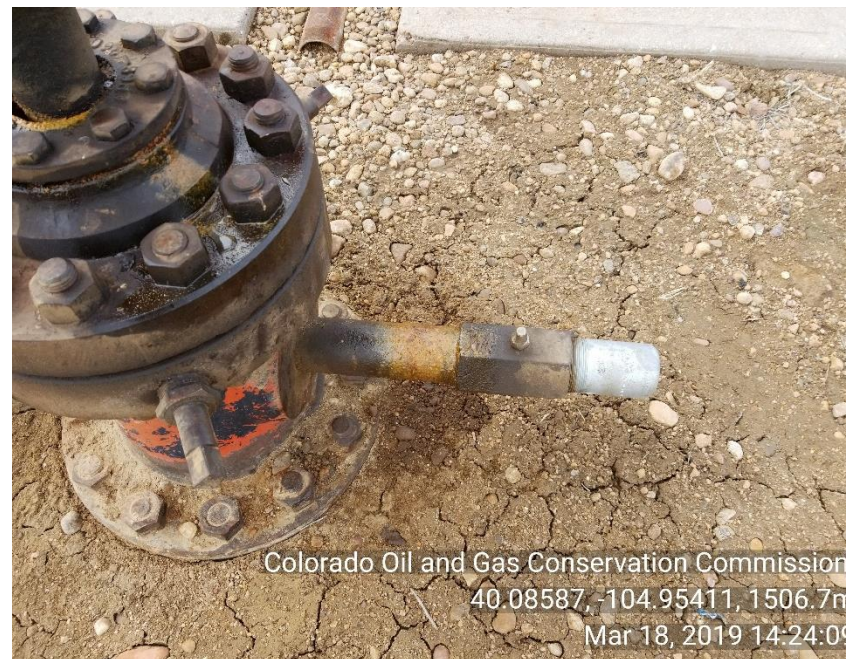
Photo 2 Mechanical issues ( 2' VLV appears to be leaking fluid) and stained soil
