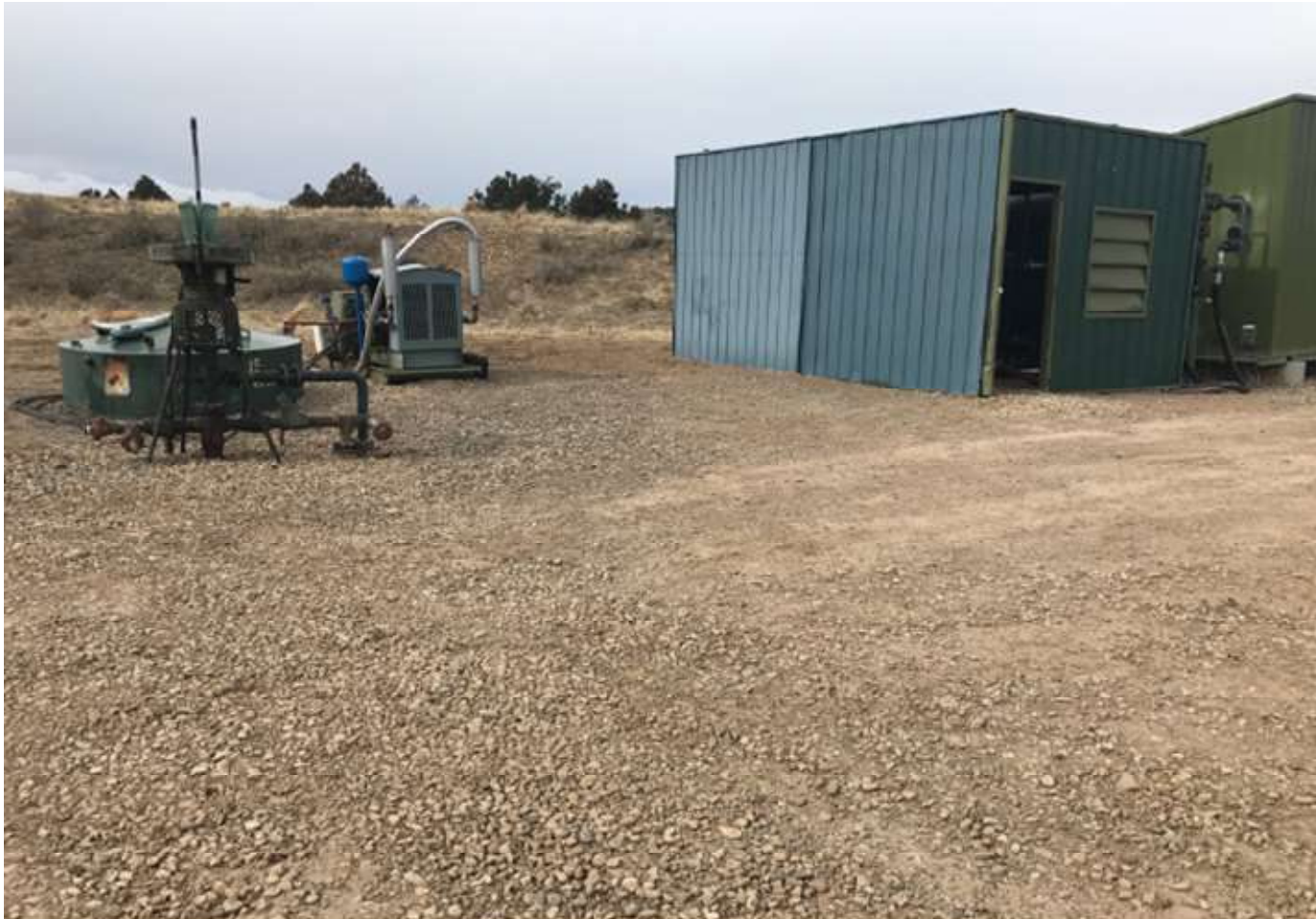
PHOTO 1: THE 15 BBL WATER TANK WILL BE PUT IN USE TO DRAIN THE FUEL SCRUBBER.
