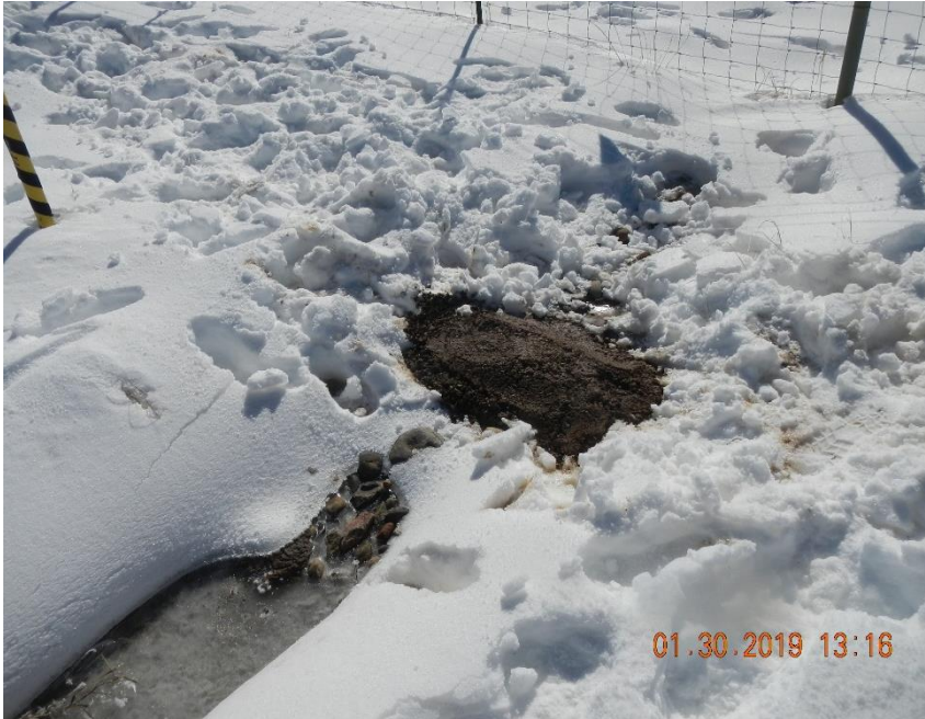
Earthen berm observed during this inspection. Reportedly stopped flow from exiting location.
