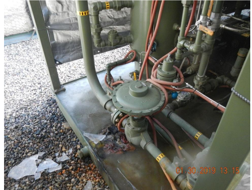
Skid mounted compressor with containment area full of ice.
