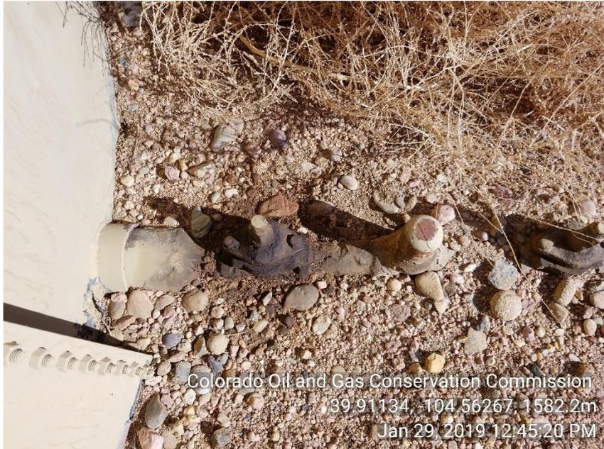
**Photo 3 stained soil load line VLV on back of west crude oil tank**
