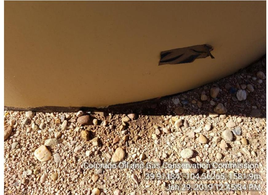
**Photo 4 Stained soil on west crude oil tank**
