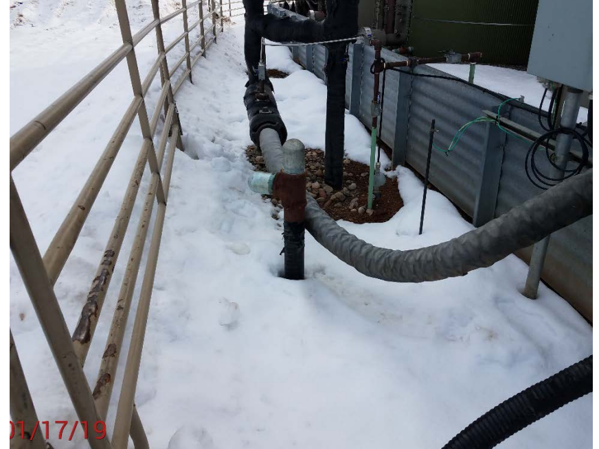
Location Photo #4, Unmarked/unused flowline near tank containment.
