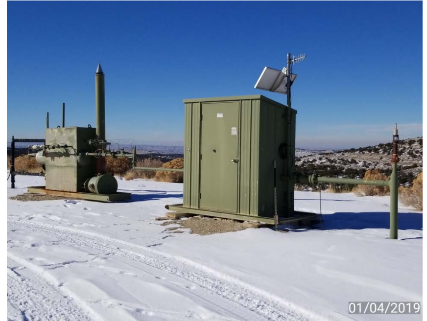
Photo 2. Separator and gas meter building.
