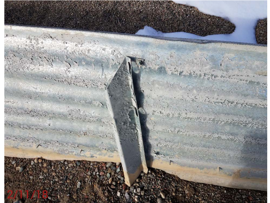
Location Photo #4, Support bracket broken.
