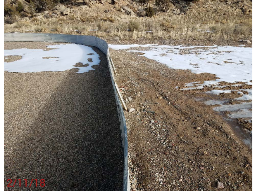
Location Photo #2, containment wall damage.
