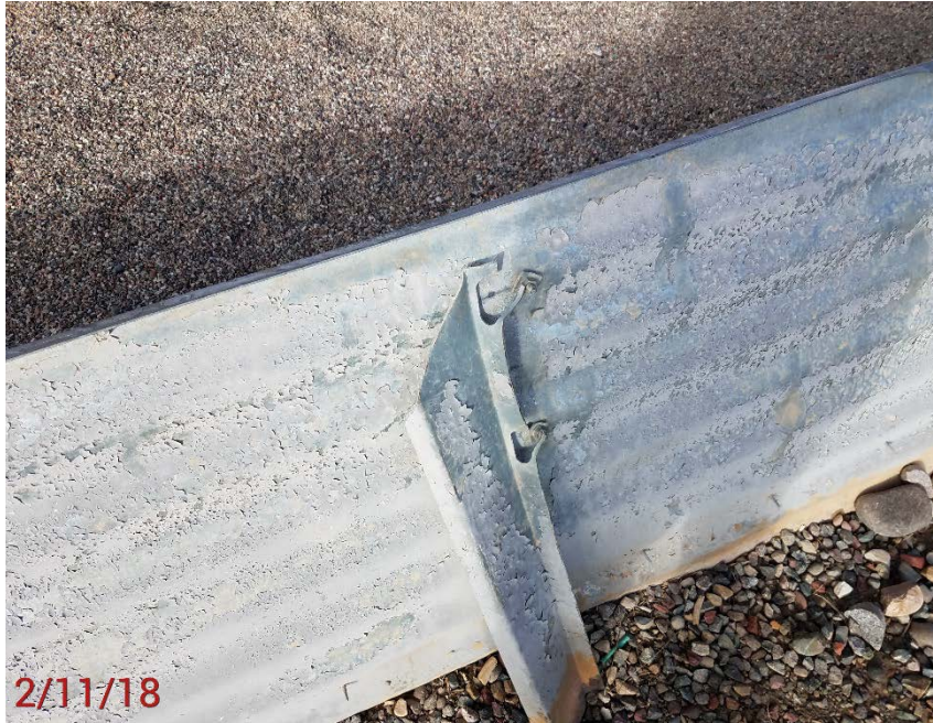
Location Photo #3, Support bracket broken.
