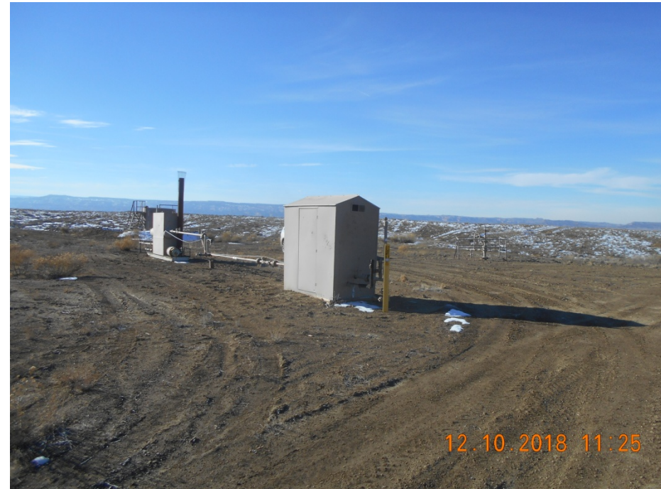
Separator and Meter housing
